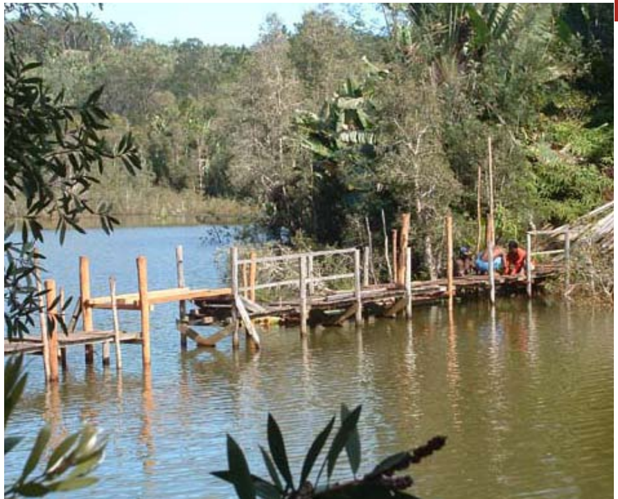
Local contractors working on one of the bridges.
